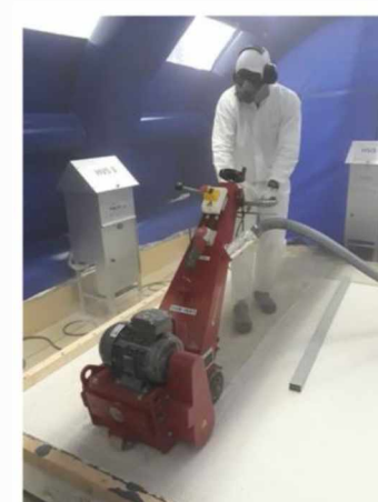
Scarifying operations of a concrete slab using a manually propelled industrial milling machine
