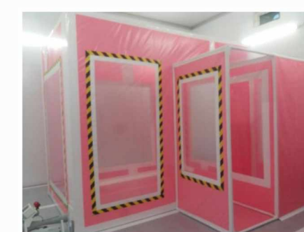
Flexible airlock in the MASSALE facility
