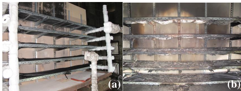
Fig. 11: Cable trays for the CT5 test. (a) before fire. (b) after fire.
