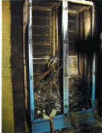
Figure 7: Cable trays after CFS-6.
