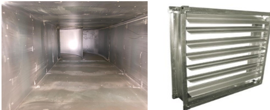
Figure 13: Inner deflector in an industrial horizontal bend CD2 (left) and ventilation damper in an open position (right)
