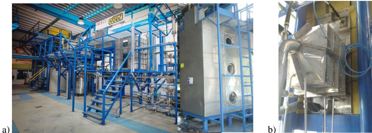
Figure 3. The VIKTORIA facility (a) and the implementation of the strainer (b)
