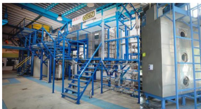
Figure 3 – The VIKTORIA Test Facility
