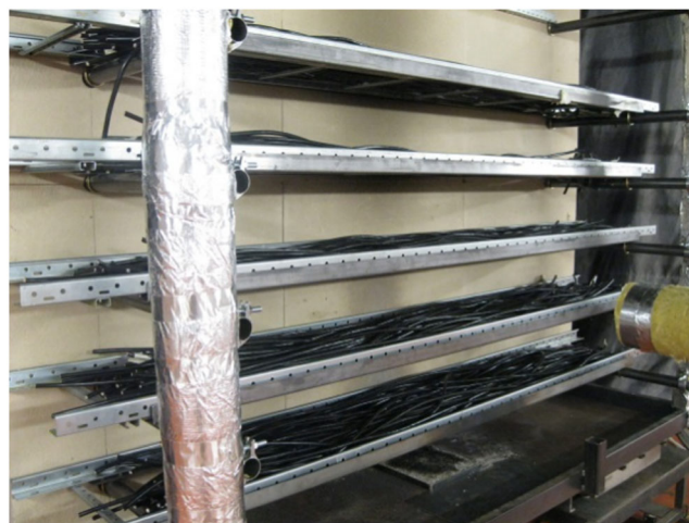
FIGURE 1 Set of cable trays used for the CFSS fire tests [Colour figure can be viewed at wileyonlinelibrary.com ]
