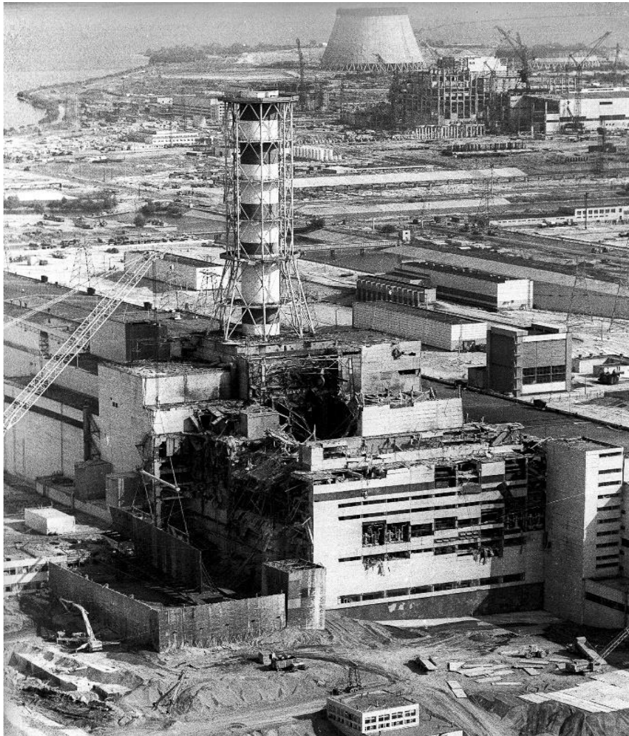
Figure I.1- The destroyed building of Chernobyl NPP, which design did not implement a containment building to enclose its reactor.
